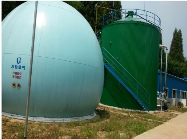
Anaerobic digester and gas storage
